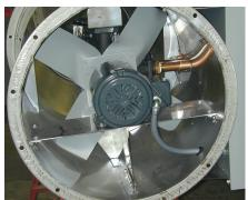
High-volume airflow with consistent velocity is provided by a heavy-duty, direct-drive axial fan.
