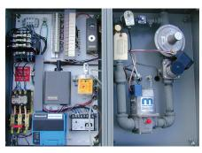
Reliability is ensured with advanced gasmanifold controls, electronic ignition, flame rod burner supervision, and diagnostic circuit check lights.
